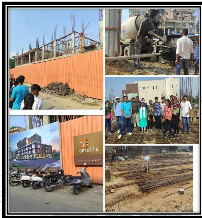
Visit to Commercial Building Construction Site: OM Elite at V.V. Nagar, 06-10-2021
